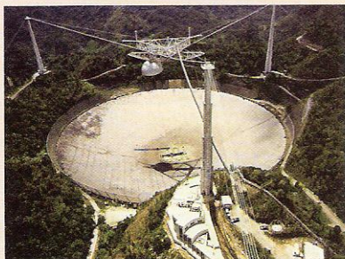
The Arecibo radio astronomy dish is located near the northern coast of Puerto Rico. Its 300-meter diameter makes the giant SETI instrument the world's largest.
