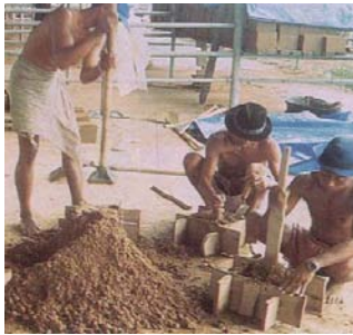
Molding using wooden bars
